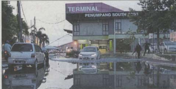
In last year's high tide incident, the sea water caused a minor flash flood outside the Pulau Ketam jetty in Port Klang. — Filepic
